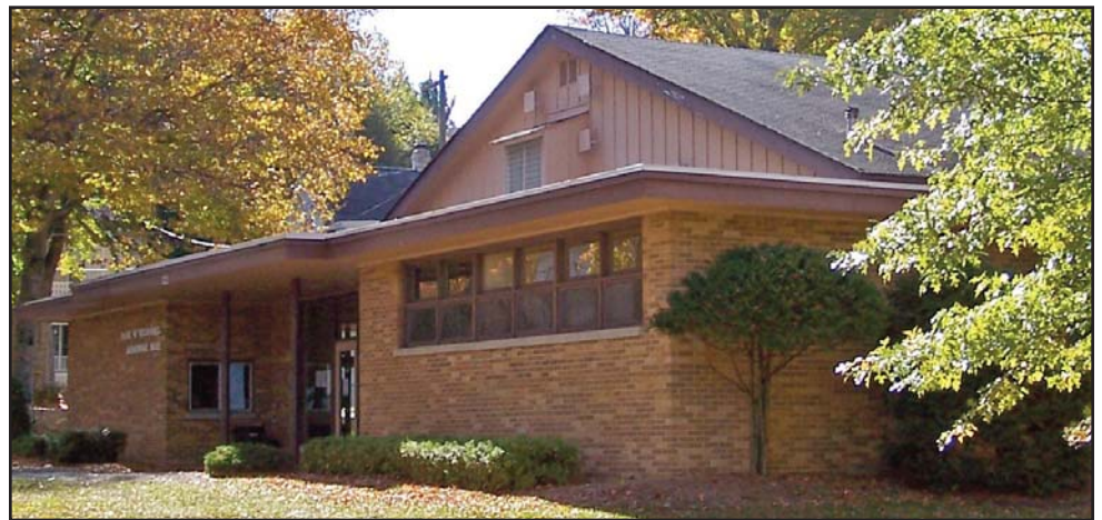
Voorhies Hall is undergoing extensive renovation. (Town Crier photo)
